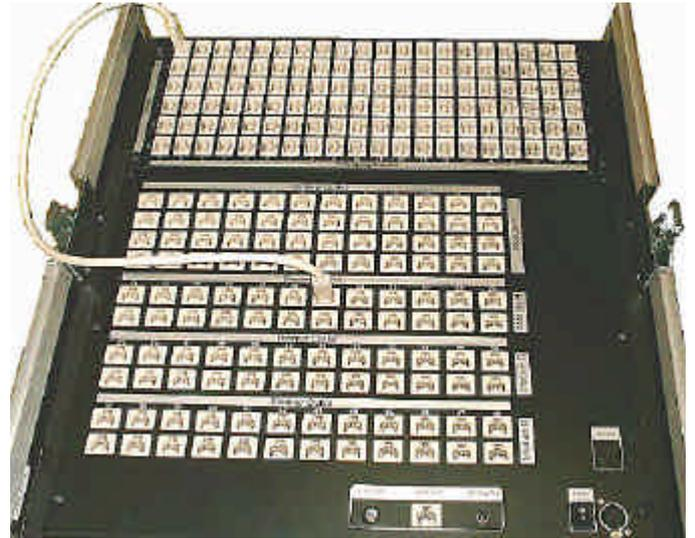
A Series patch requires two loads to be connected to work, this as the 2 loads will be wired in series with each other to allow the use of 110V lamps. The first bay allows two sets of loads to connected (thus four loads are needed)
